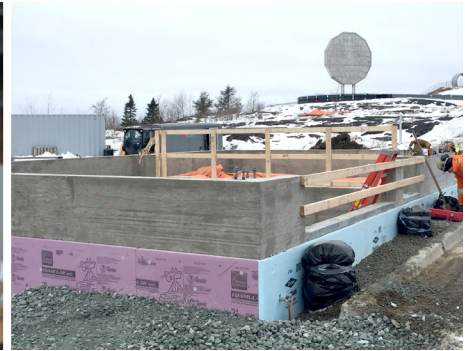
Dr. Dean Millar's project under construction at Dynamic Earth
